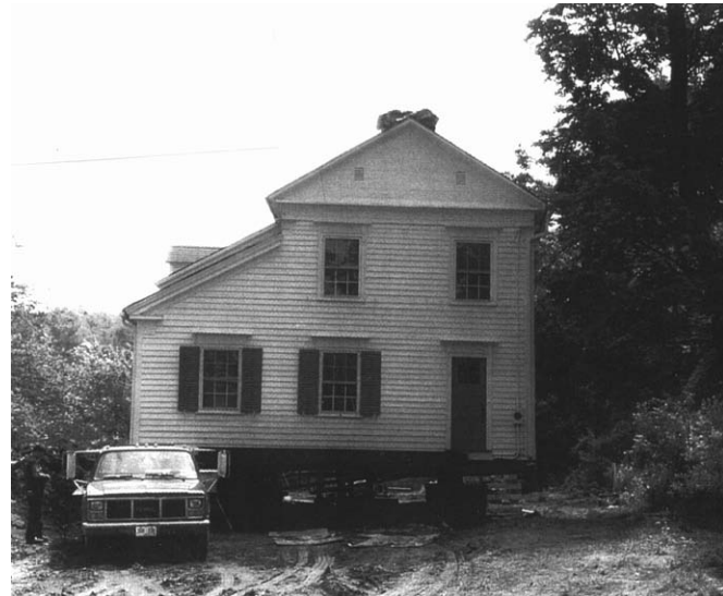
The old toll house being moved.
