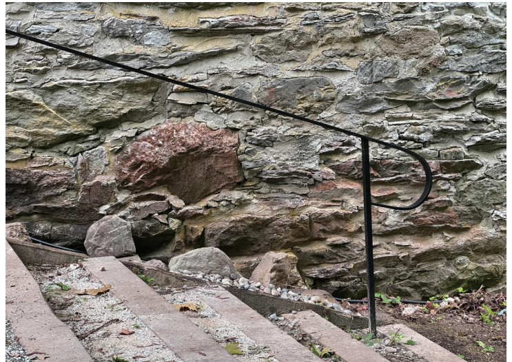
IRON RAILING INSTALLED
